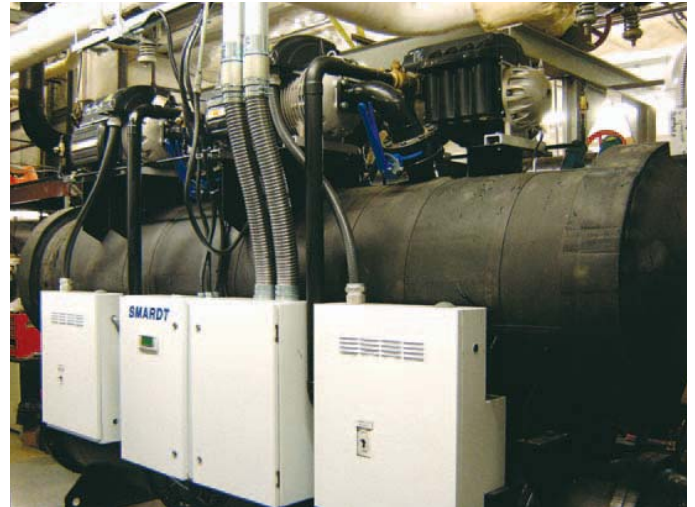
The Smardt 350 tr water cooled chiller installed at the Sears mall at Halifax, Nova Scotia has been delivering reliable energy savings since the day it was commissioned.
